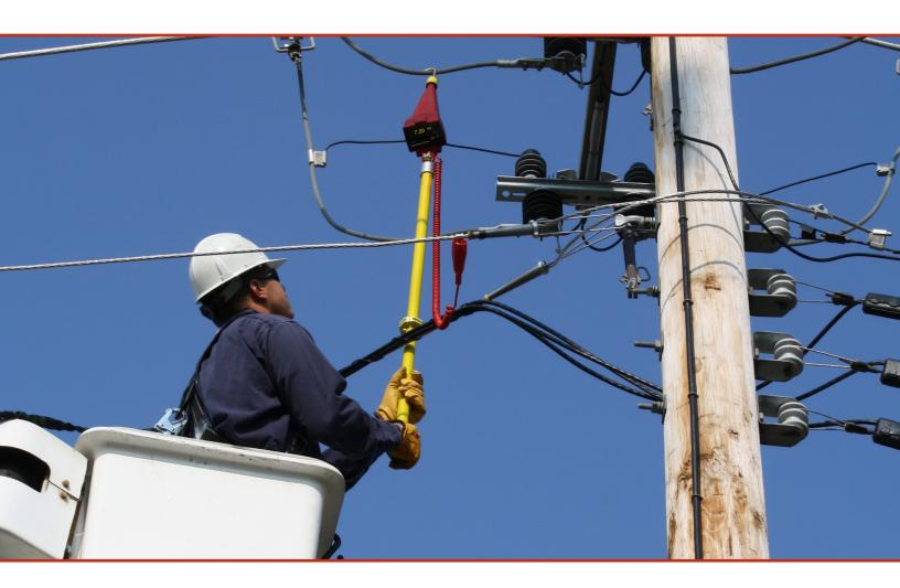
The single stick digital voltmeter, model SVM-25, is a highly accurate one stick voltmeter with a large digital display, peak hold and capacitive test point mode.
